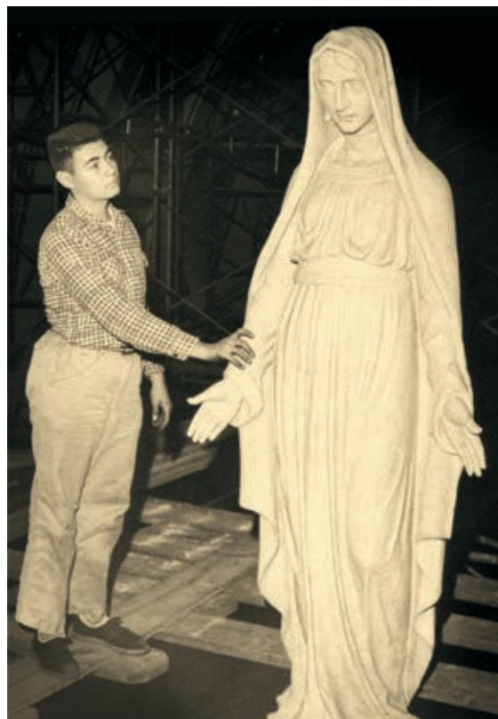
Joseph Kolosky, son of photographer Basil Kolosky, with Our Lady during 1953 dome restoration work.
