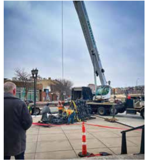
Sculpture Installation, March 29, 2024
