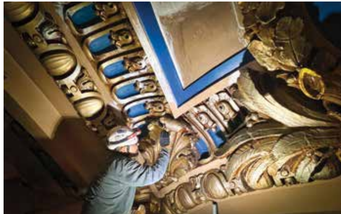
Plaster worker on scaffolding
